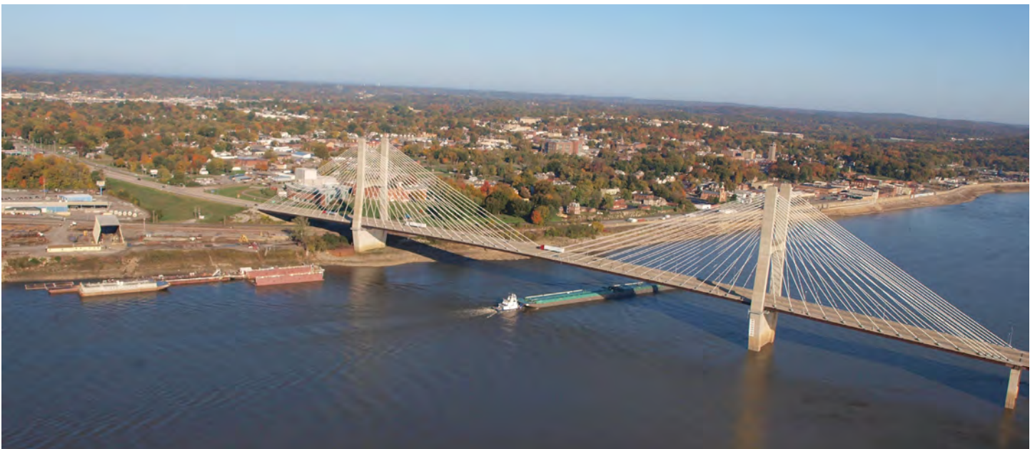
Bill Emerson Memorial Bridge
