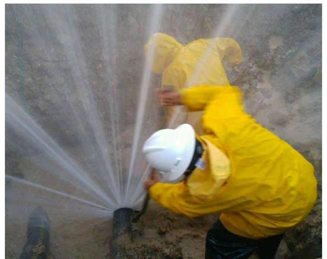
Water Line Repair
