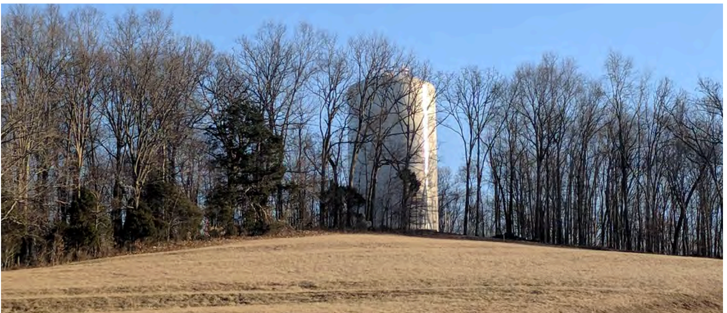
LaSalle Water Tank
