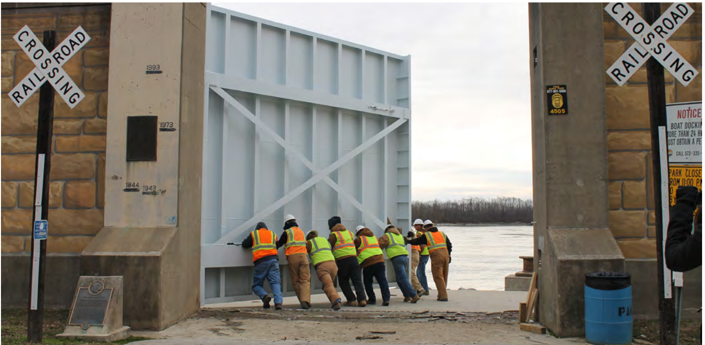
Reopening the Themis Street Flood Gate
