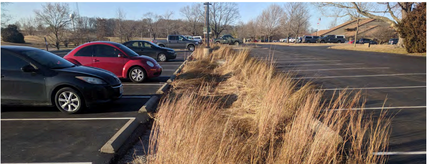
Green infrastructure in the Cape Girardeau Conservation Nature Center parking lot
