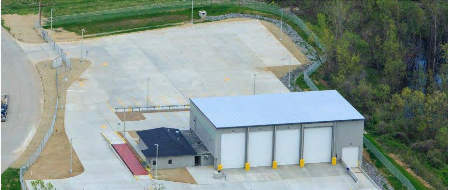
Exterior of Transfer Station
